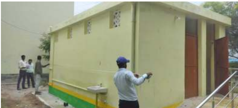
Construction of Community Toilet.
