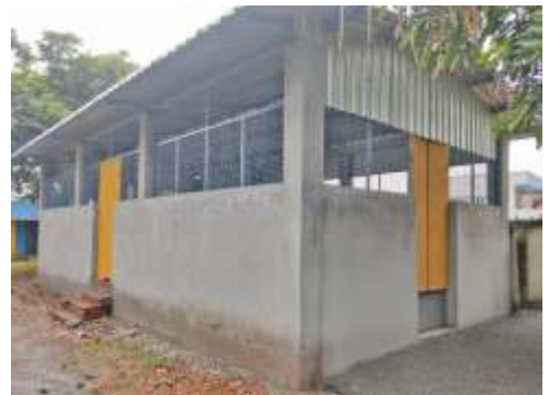
Construction of Dining Centre for students
